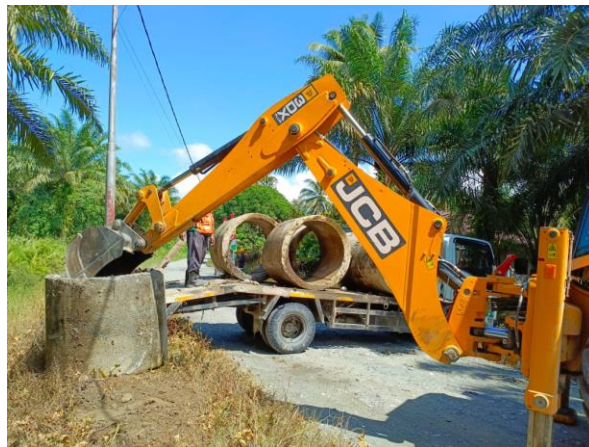
Bridge construction to connect the access to public cemetery location
